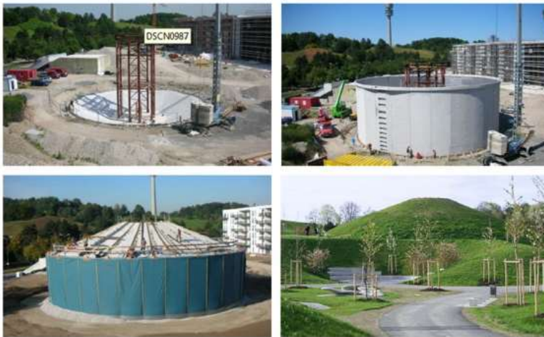
5700 m 3 heat store 2900 m 2 solar thermal, Munich 2007
